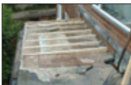
Firrings fixed to a flat roof to aid run-off
